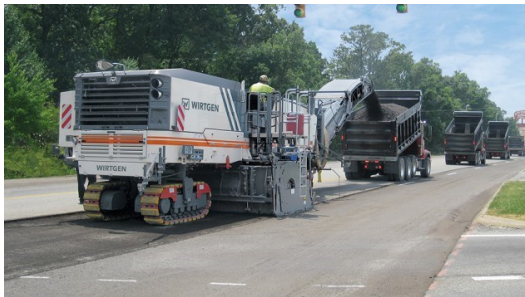
Cold milling will remove the upper section of the existing street surface.
